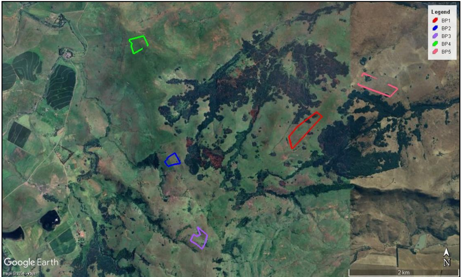
FIG. 2: AERIAL OVERVIEW OF THE DEVELOPMENT
